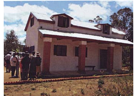
The new grain store and skills centre at Vohitromby
